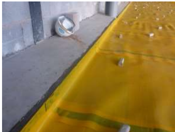
Plate 3: Gas membrane installation up to existing internal wall
