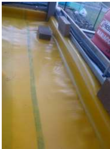
Plate 2: Gas membrane installation up to external wall
